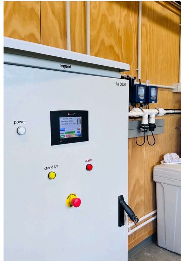
Pictured above: Envirolyte generator unit, generating ANK Neutral Analyte onsite
